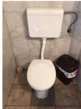
2.1 & 2.2. beach toilets are upgraded
